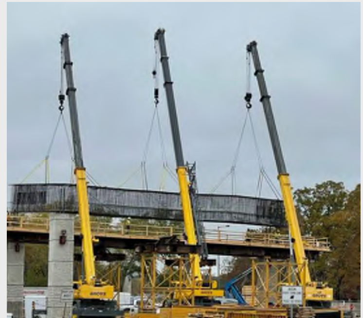
Three-crane lift of US 290 mainlane bent cap
